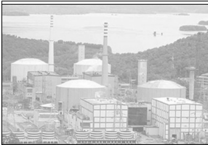
Kaiga Power Plant
